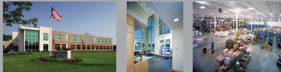
Our 200,000 sq. ft. manufacturing facility in Melville, NY.
